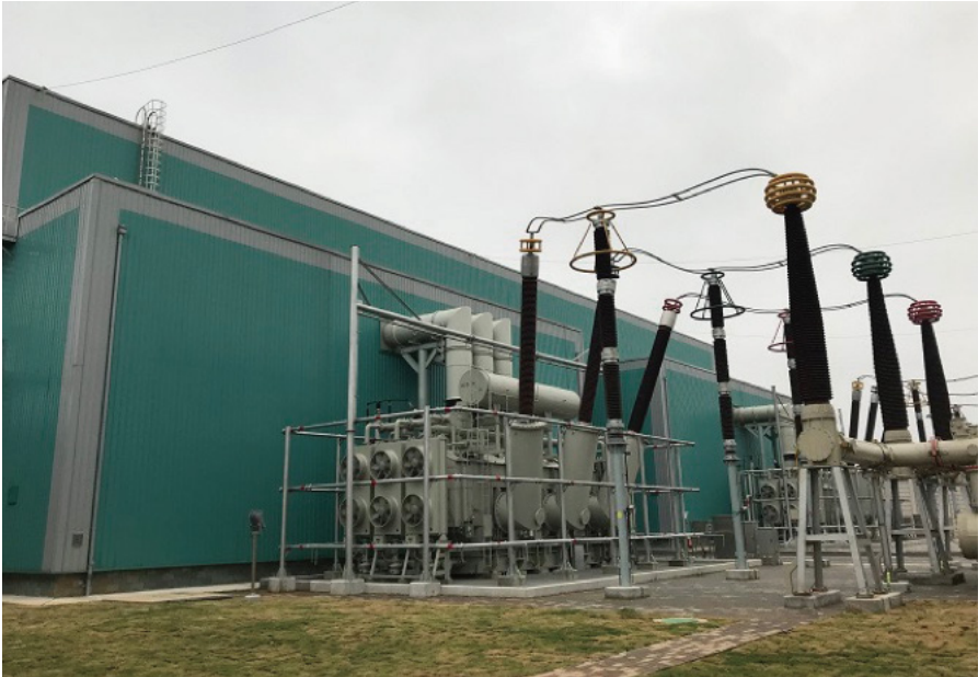
Synchronous condenser picture taken on site
